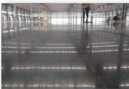
Concrete Polishing and Densification
