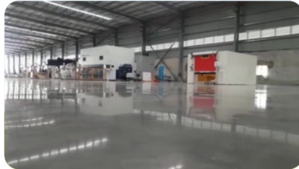
Bosch - Warehouse, Chennai
