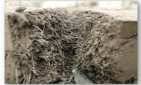
Steel Fiber Reinforced Concrete Flooring
