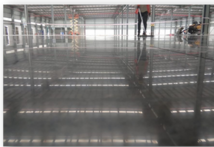
Concrete Polishing and Densification
